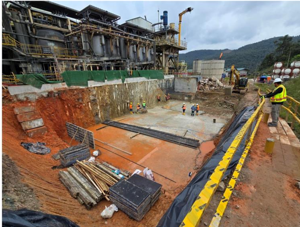
Jameson cell foundation excavation
