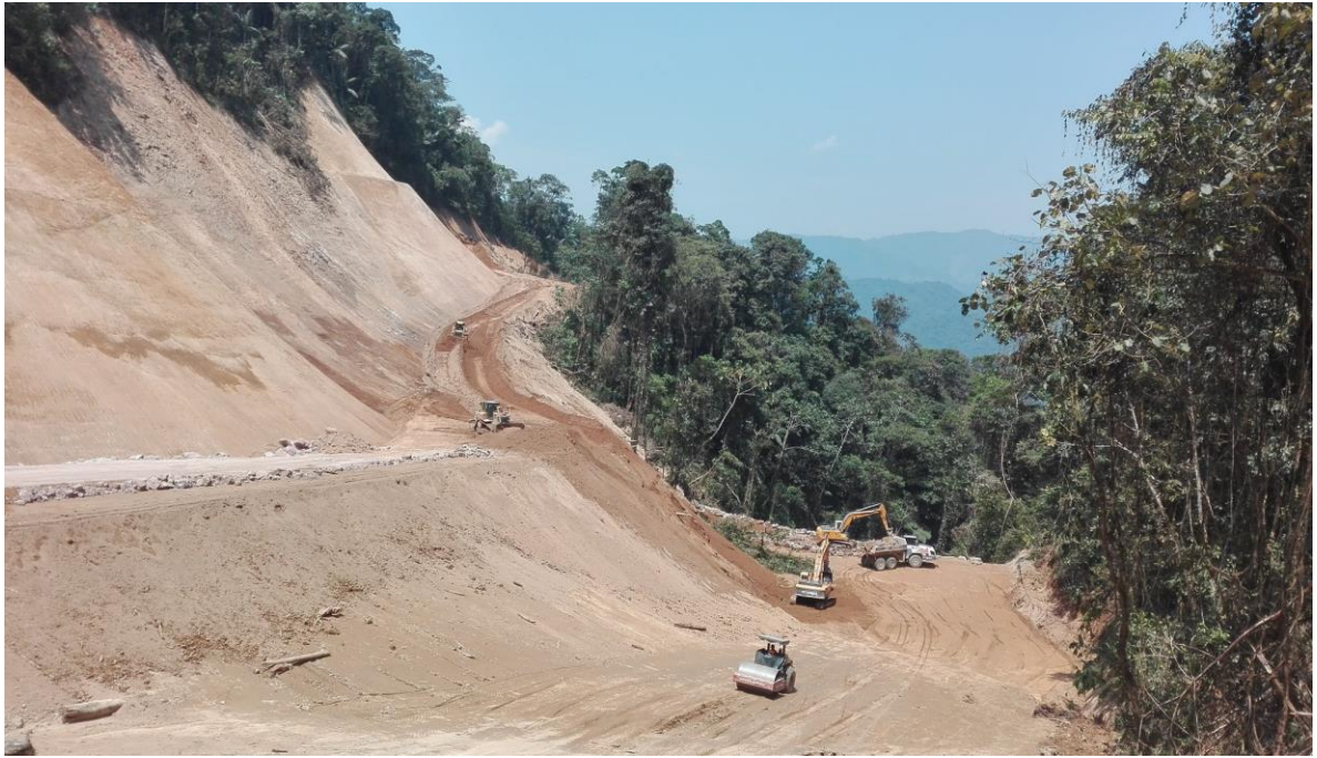
Figure 6. Construction of the Tailings Storage Facility ongoing
