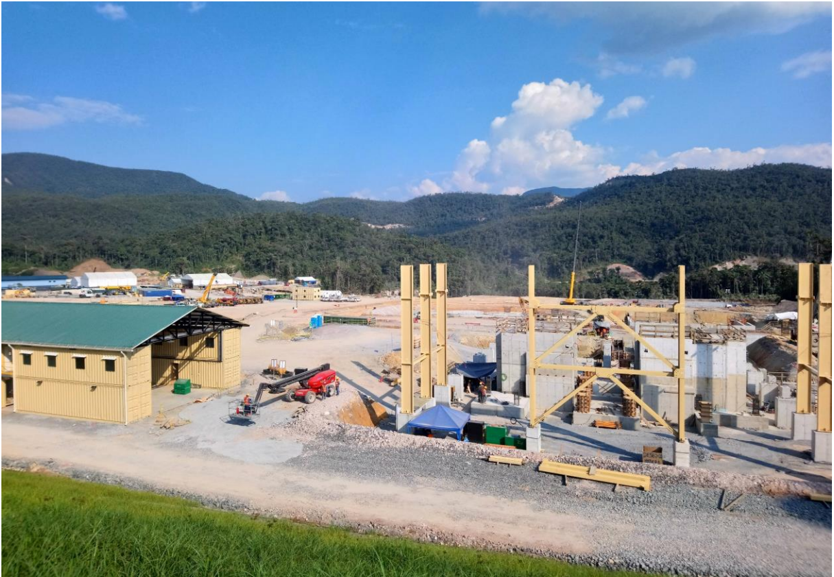
Figure 4. Carbon-in-leach tank foundations
