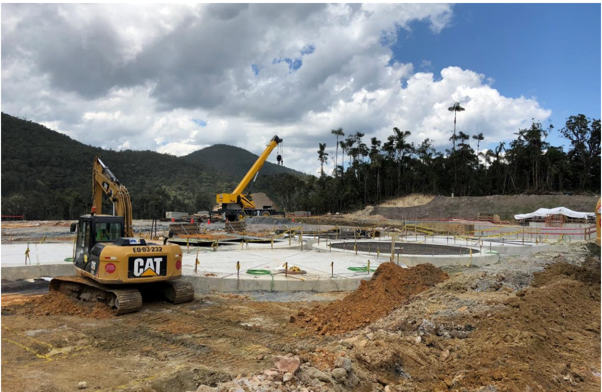
Figure 4. Carbon-in-leach tank foundations
